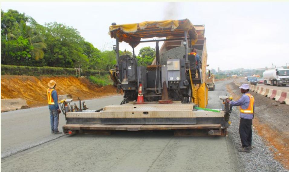
*Laying the stone base on a section of the Abuja-Kano Road.*
